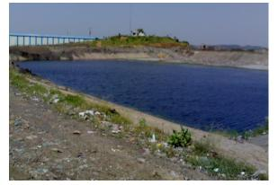
commissioning of new site, the waste started to transport here for processing as well as landfill. This site at village Kedarpur developed by M/s AKC Developers have disposal as well as leachate collection tank of HDPE liner to avoid ground water contamination.
